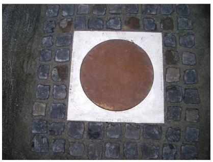
Installation of the aluminium mount including the round steel plate (as a kind of place holder) at first.
