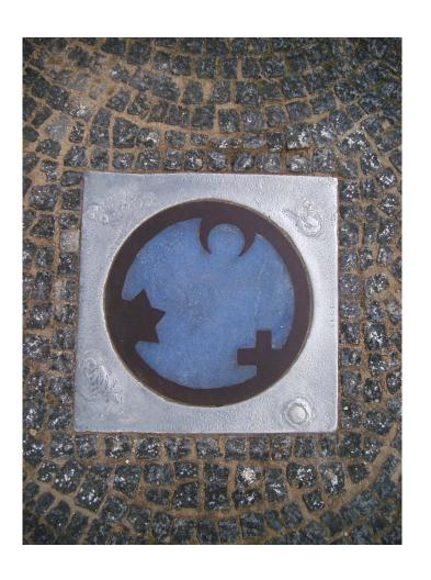
With the Ground inlaid work the Angel of Culture will be embedded into the ground in form of a steel ring, with blue coloured special concrete inside of an aluminium frame.
